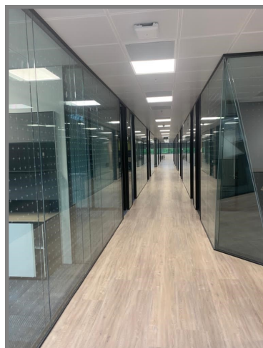
503lm of double glazed partitions including bespoke corner sections and over 100 double glazed doors.
